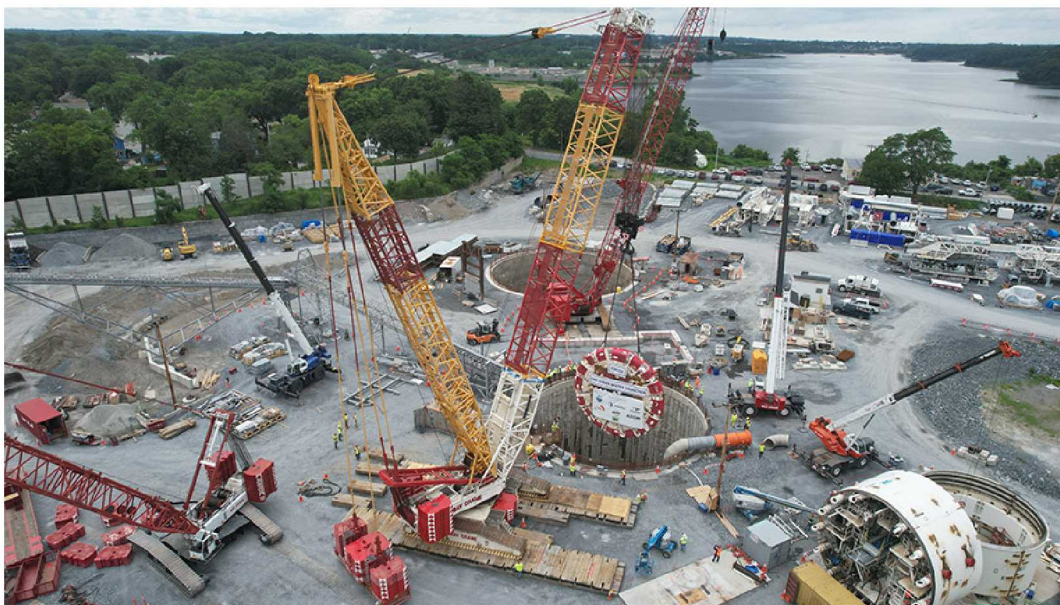
NBC CSO III tunnel construction
