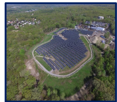
North Prov. Landfill 2.60 MW North Providence, RI Power Off-Taker: Town of North Providence
